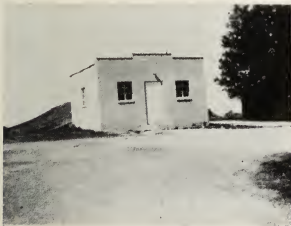
Rock City Water System Pumping Station
