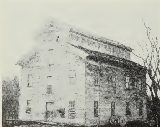
Addams' Mill, Cedarville. Occupied a site just across the road from the present site of the John H. Addams house, it was later moved and rebuilt into the barn now standing at the Addams homestead. It was one of the largest mills in the county and was run by the father of Jane Addams.
